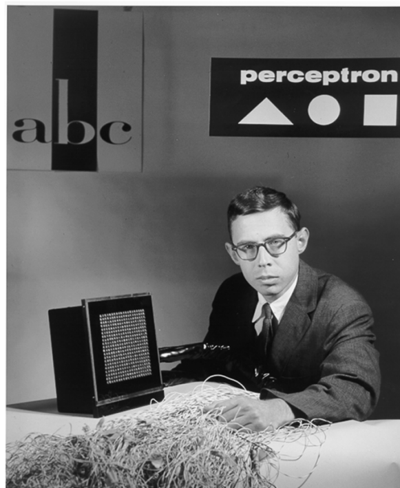
Rosenblatt's Mark I Perceptron, an analog machine operating with a 20x20 photocell array (Source: Computer History Museum)
